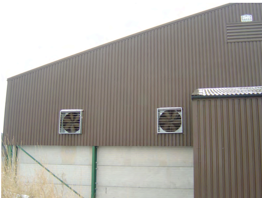
Hydor HV Fans installed in the Grain Store
